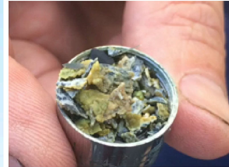
Tap aerator debris
